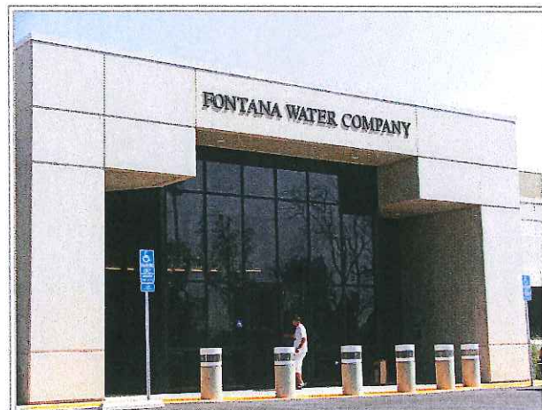
The City of Fontana and the Fontana Water Company have signed a joint recycled water project agreement that will take highly treated wastewater and use it on landscaped areas around the city, a move which is expected to save more than 600 million gallons of fresh drinking water each year.
