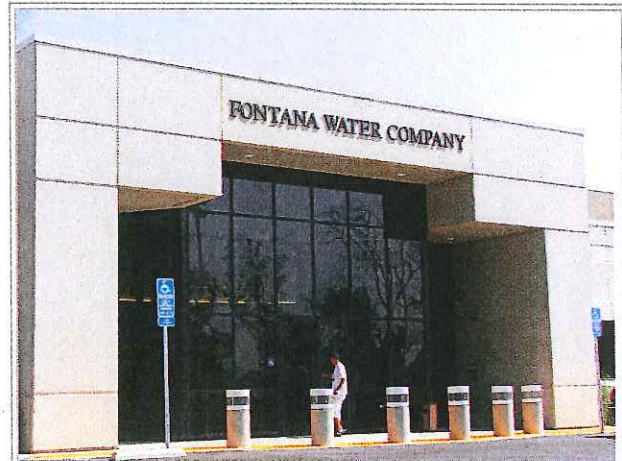
The City of Fontana and the Fontana Water Company have signed a joint recycled water project agreement that will take highly treated wastewater and use it on landscaped areas around the city, a move which is expected to save more than 600 million gallons of fresh drinking water each year.
