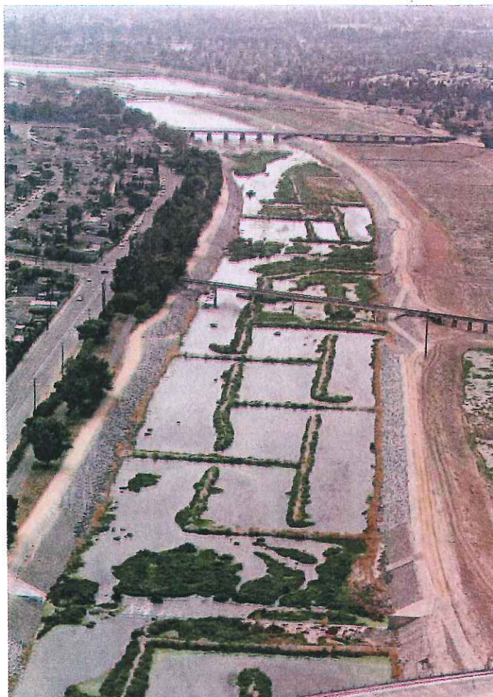
Basins capture water on the Santa Ana river, allowing it to percolate into the aquifer underground. Register file photo by Jebb Harris.
