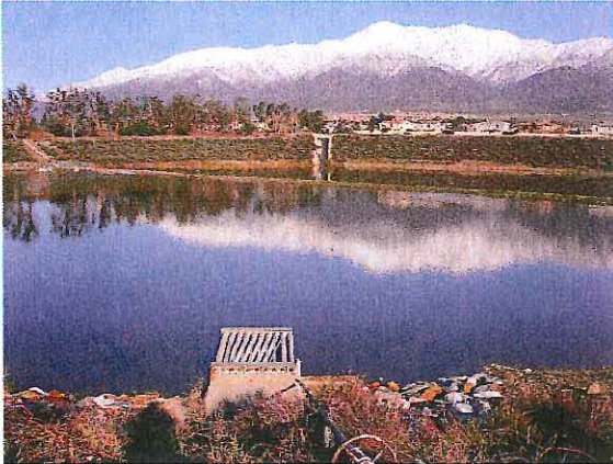
Recharging the Chino Basin Groundwater at Victoria Basin
