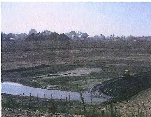
Turner Basins Recharge Expansion Project Excavation Milliken Grade Separation Stockpiles in Background
