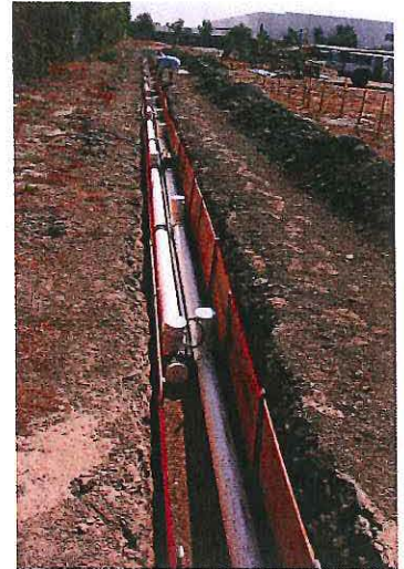
Horizontal Extensometer Construction
