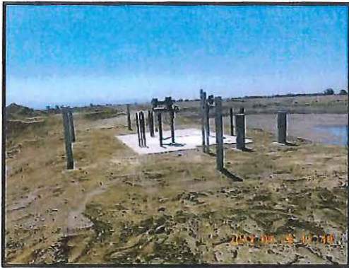
Completed Junction Structure
