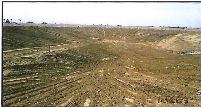
Completed new south basin
