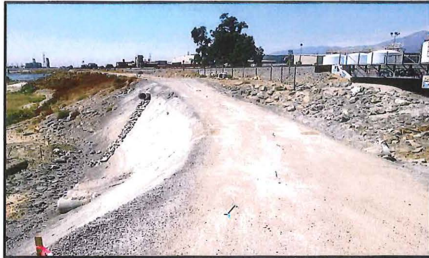
Completed access road leading to the north side of Hickory Basin
