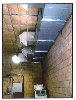
Installed ceiling insulation and AC air ducting
