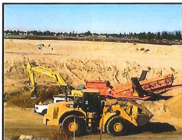
New north basin (Turner 4b) – grading/hauling in progress
