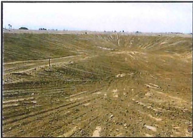
Completed new south basin (Turner 4c)
