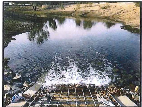
Completed new outlet basin north of Gausti Park (Turner 8)
