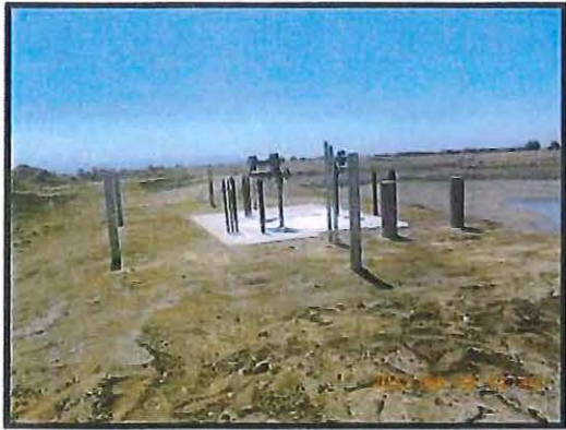
Completed junction structure
