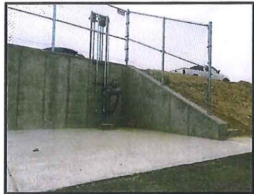
Completed valve and structure
