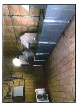
Installed ceiling insulation and AC air ducting
