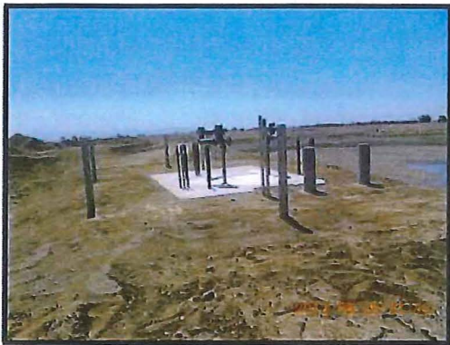
Completed junction structure
