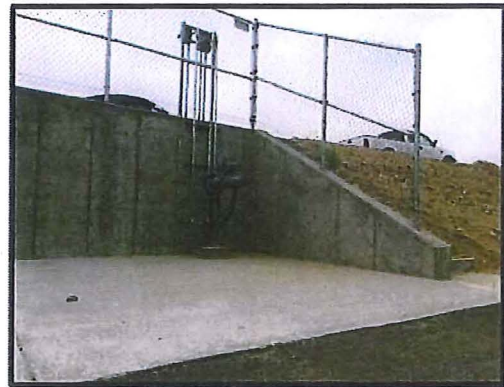
Completed valve and structure
