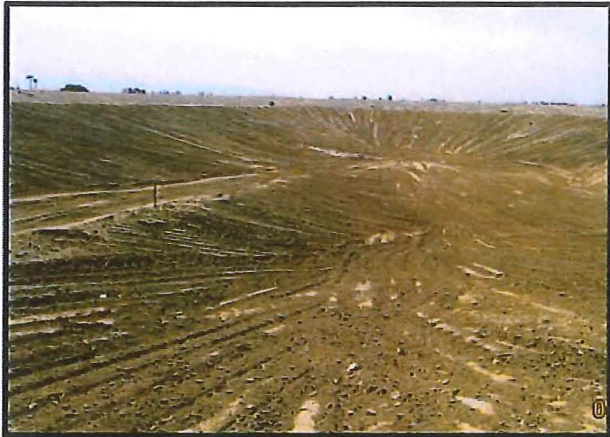
Completed new south basin (Turner 4c)
