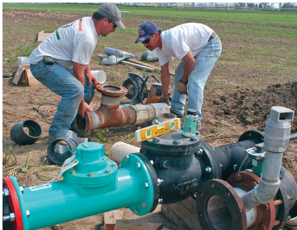
Crews installing meters for the groundwater monitoring program.
