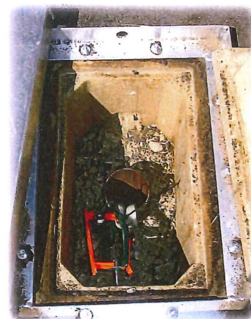
Monitoring Well with a Transducer
