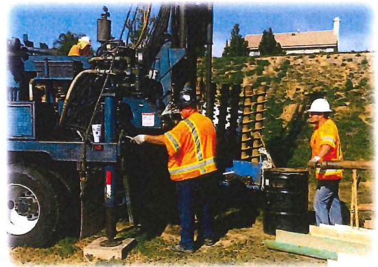
PBHSP PB-4 Well Drilling
