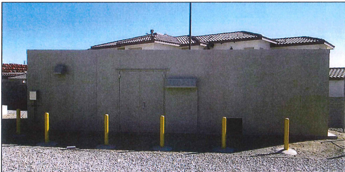
Completed installation of sound enclosure (facing south)
