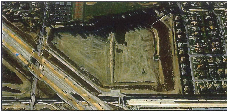
Aerial of Victoria Basin
