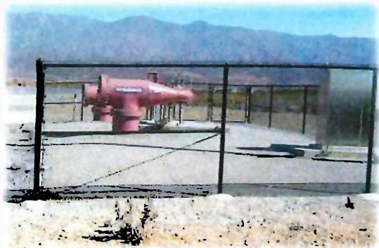
Recycled Water Line at the San Seavine Basins
