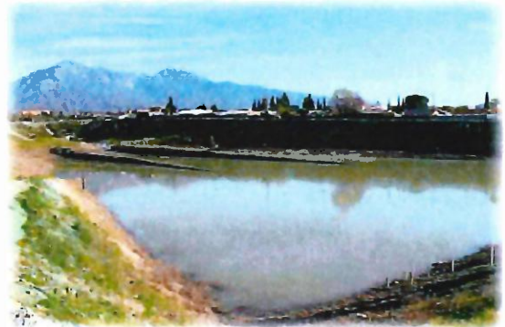
Montclair 1 Basin after a rain storm.
