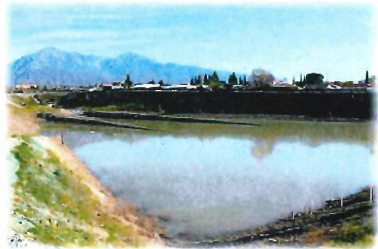
Montclair 1 Basin after a rain storm.
