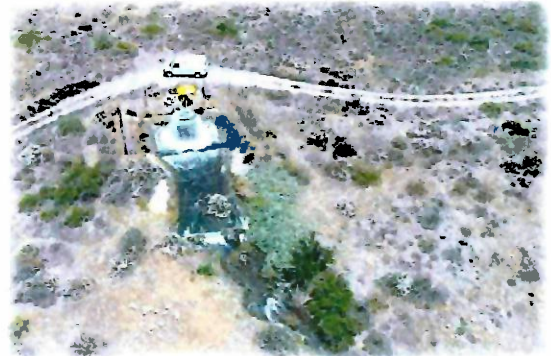
MWD Delivery North of the San Sevaire Basins.
