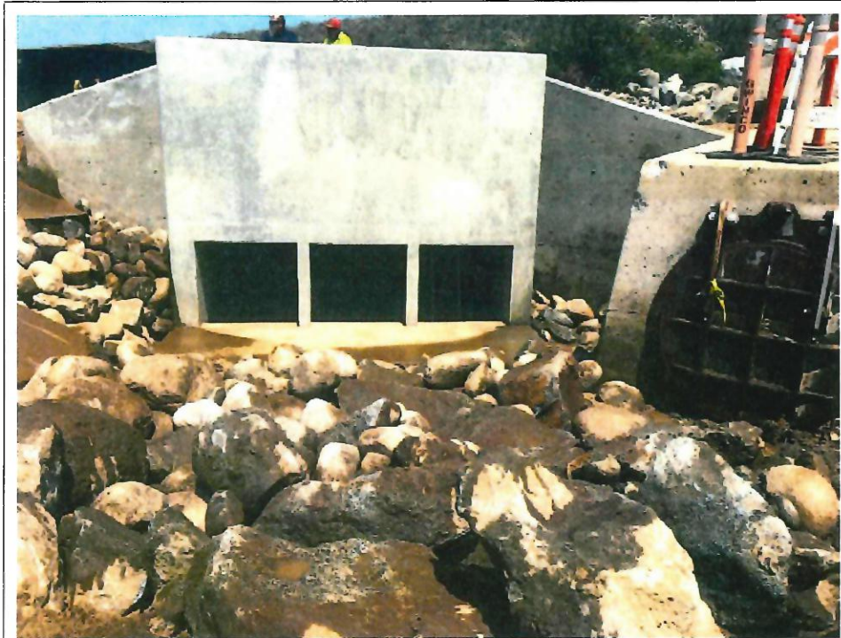
Installed new stormwater inlet structure
