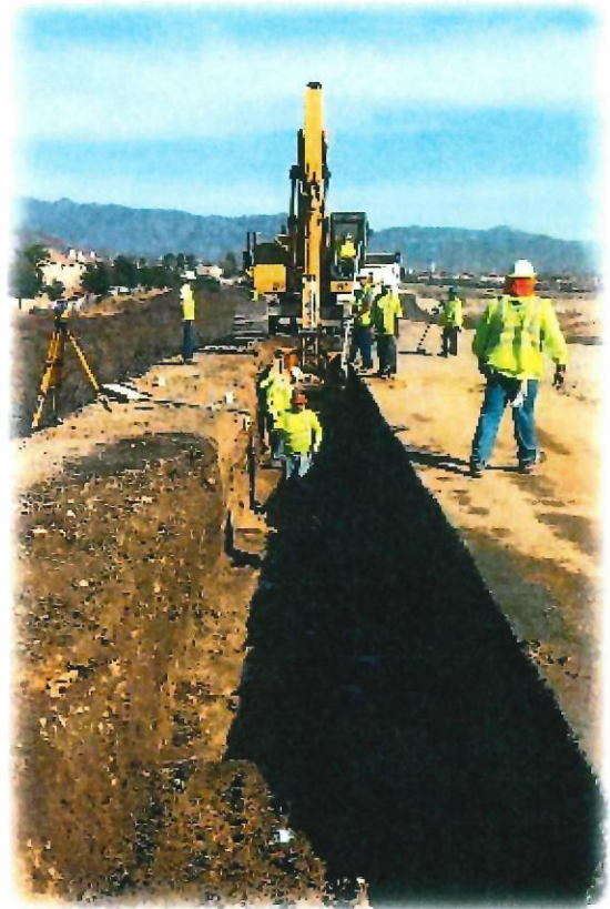
Trenching for a Pipeline at San Sevaime Basin
