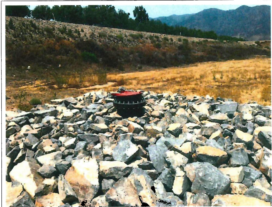
Completed Stormwater Outlet Structure in Basin 3
