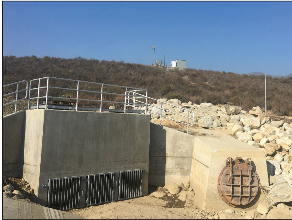
Completed Stormwater Inlet (Pump Station) – Adjacent to Existing Outlet Pipe (right)
