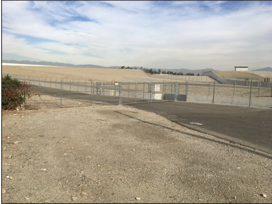
Near Jurupa Path of New 30-Inch Pipeline
