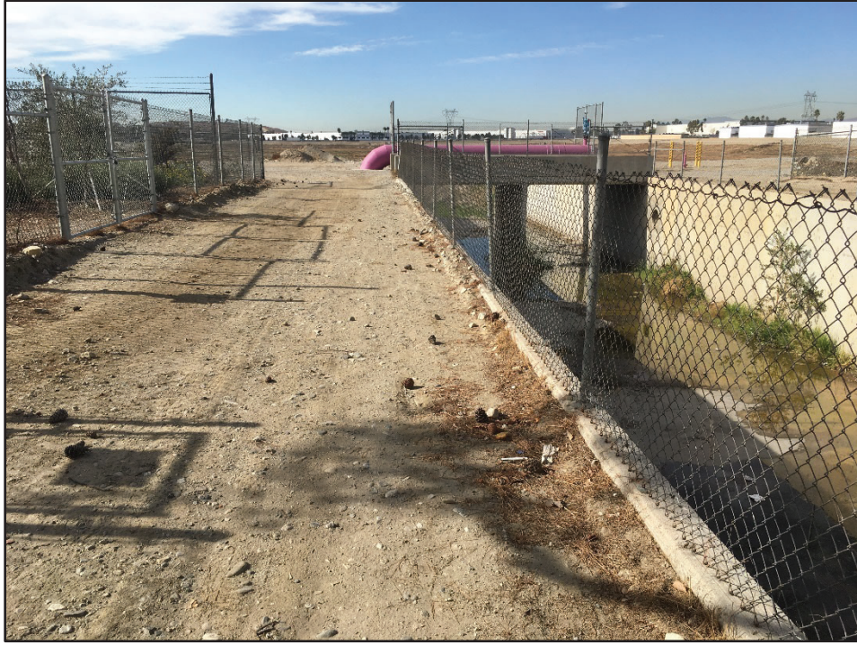
Near Wineville - Path of New 30-Inch Pipeline
