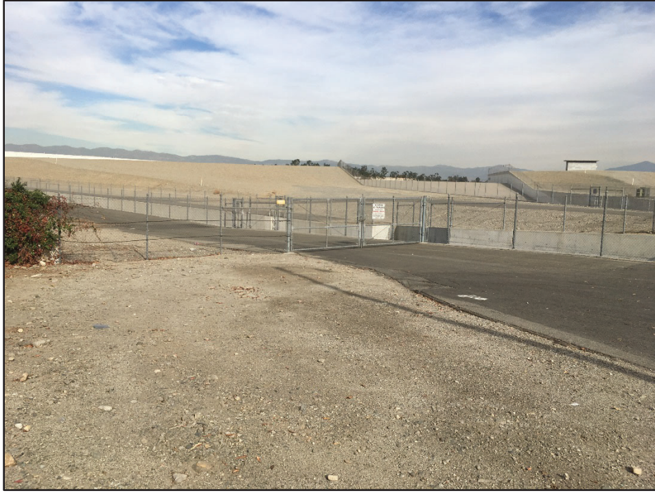
Near Jurupa Path of New 30-Inch Pipeline
