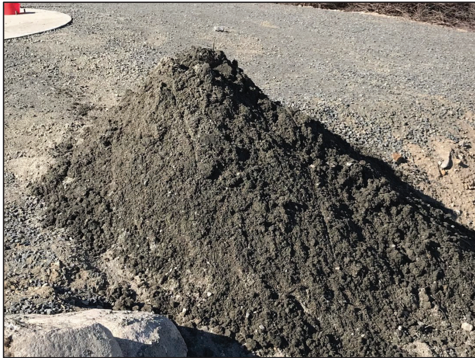
Removed Alluvial Deposits within the Pump Station Wet Well (less than 1 cubic yard)
