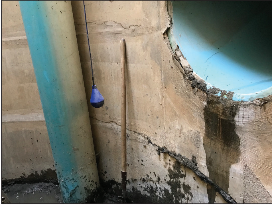
Recent Access into Pump Station Wet Well for Cleaning
