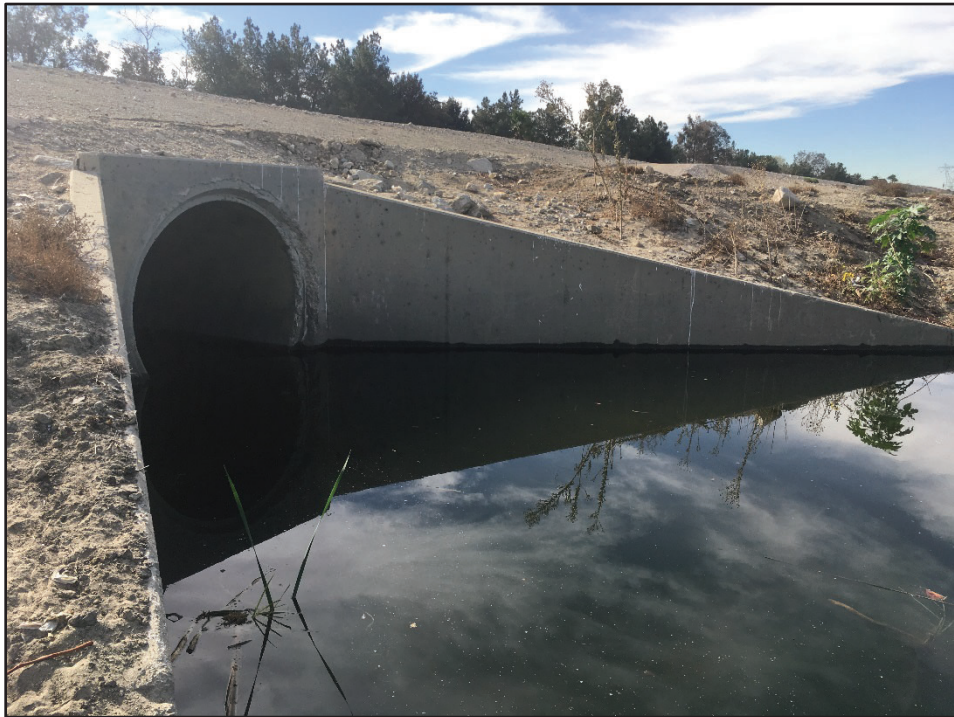
Wineville – Existing Basin Outlet
