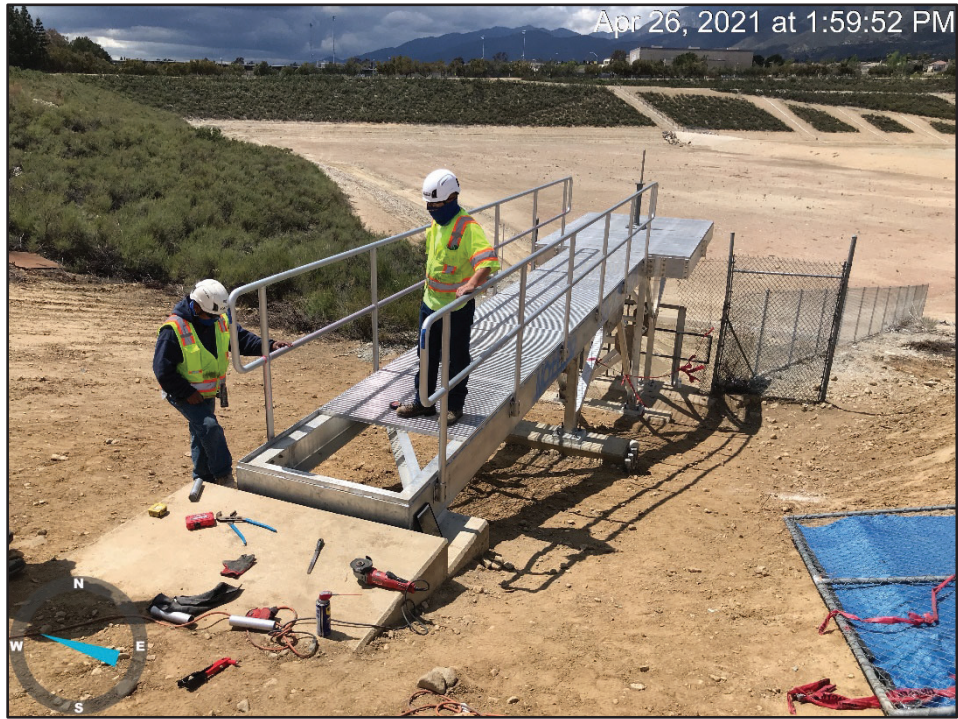
Lower Day – New Catwalk for Cell 3
