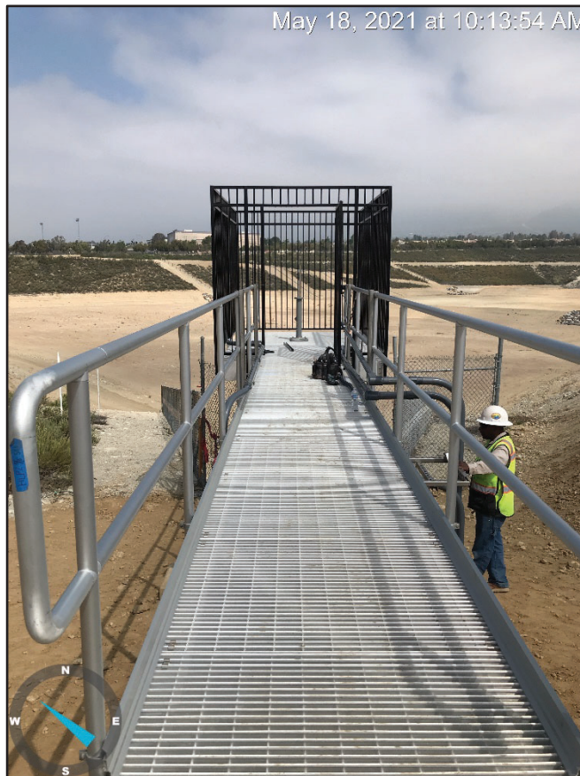
Lower Day – New Catwalk for Cell 3
