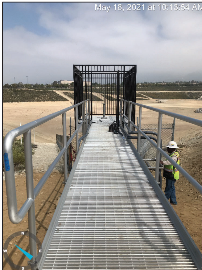
Lower Day – New Catwalk for Cell 3
