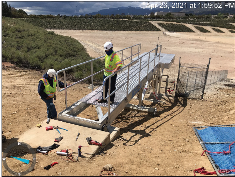
Lower Day – New Catwalk for Cell 3
