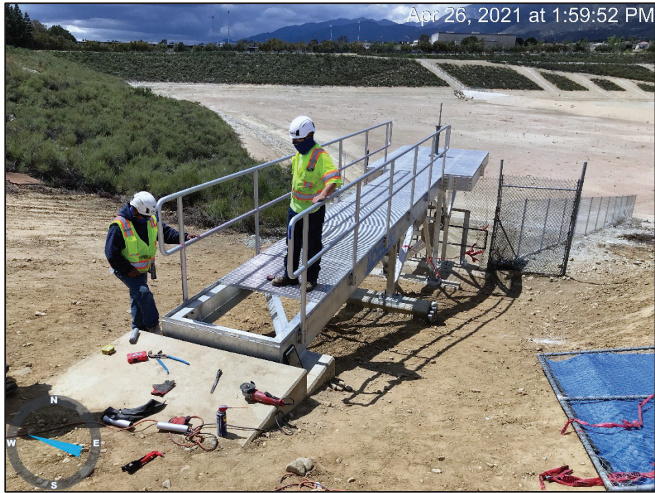
Lower Day – New Catwalk for Cell 3
