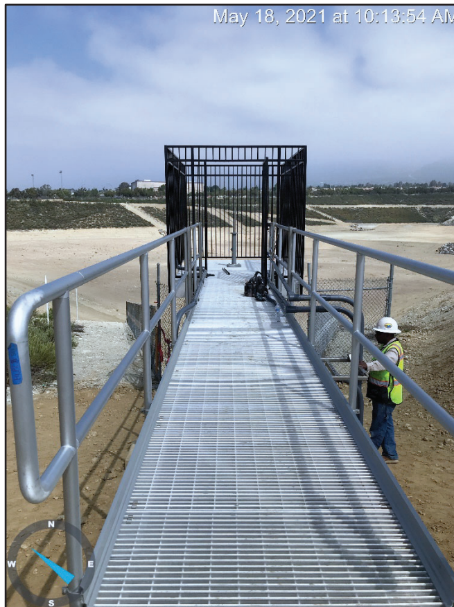
Lower Day – New Catwalk for Cell 3
