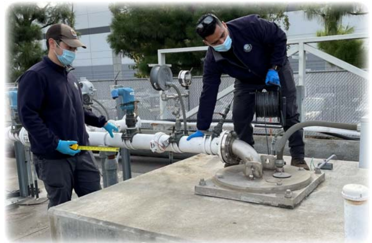
Watermaster Field Staff Measuring Groundwater Level at a CDA Well
