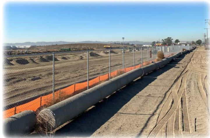
Development and Urbanization Continues Near The Chino Airport
