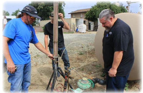
Meter Vendor Testing a Well's Inline Meter for Accuracy
