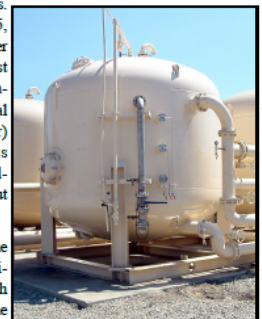
Figure 2: GAC Water Treatment System
