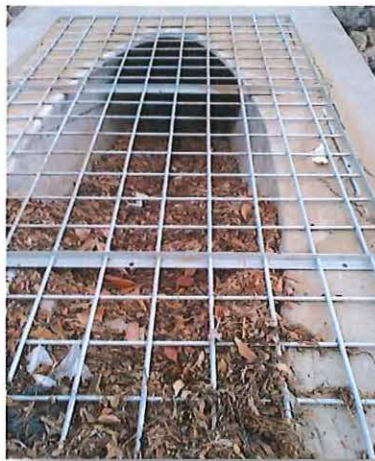
Installed 60-inch connection pipe into Basin 8
