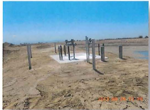
Completed Junction Structure with gates
