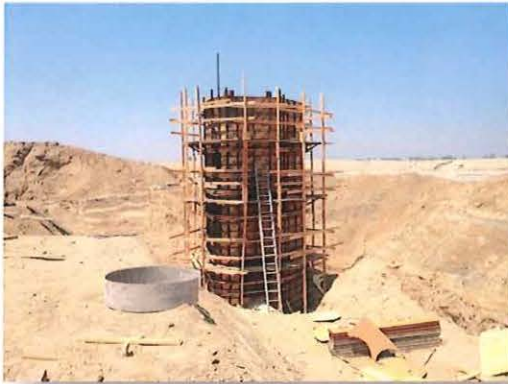
Construction of Junction Structure
