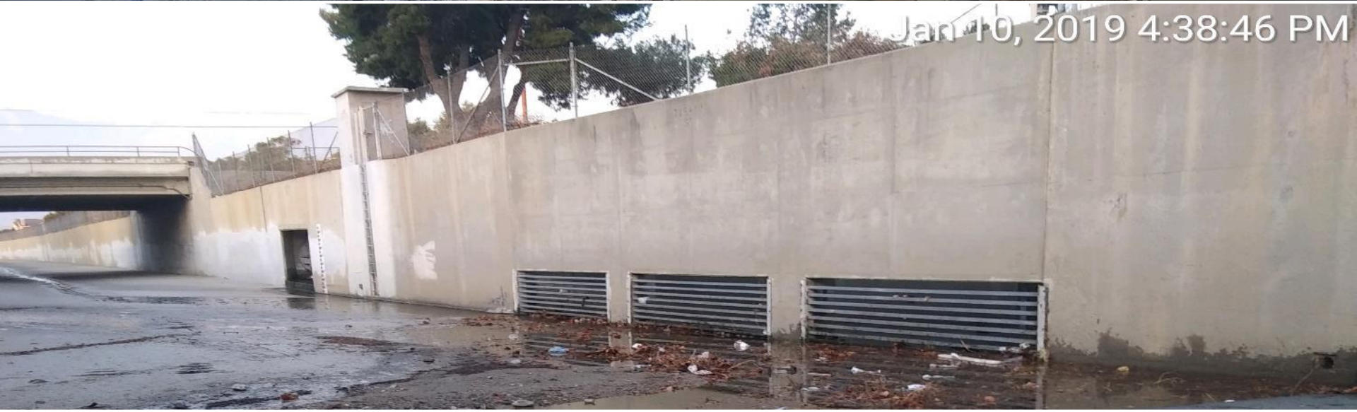
AFTER STORM RESPONSE TURNER 1 INLET CLEANING
