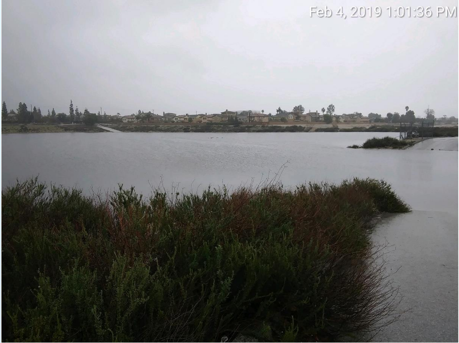
Turner 1 basin with water over road.
