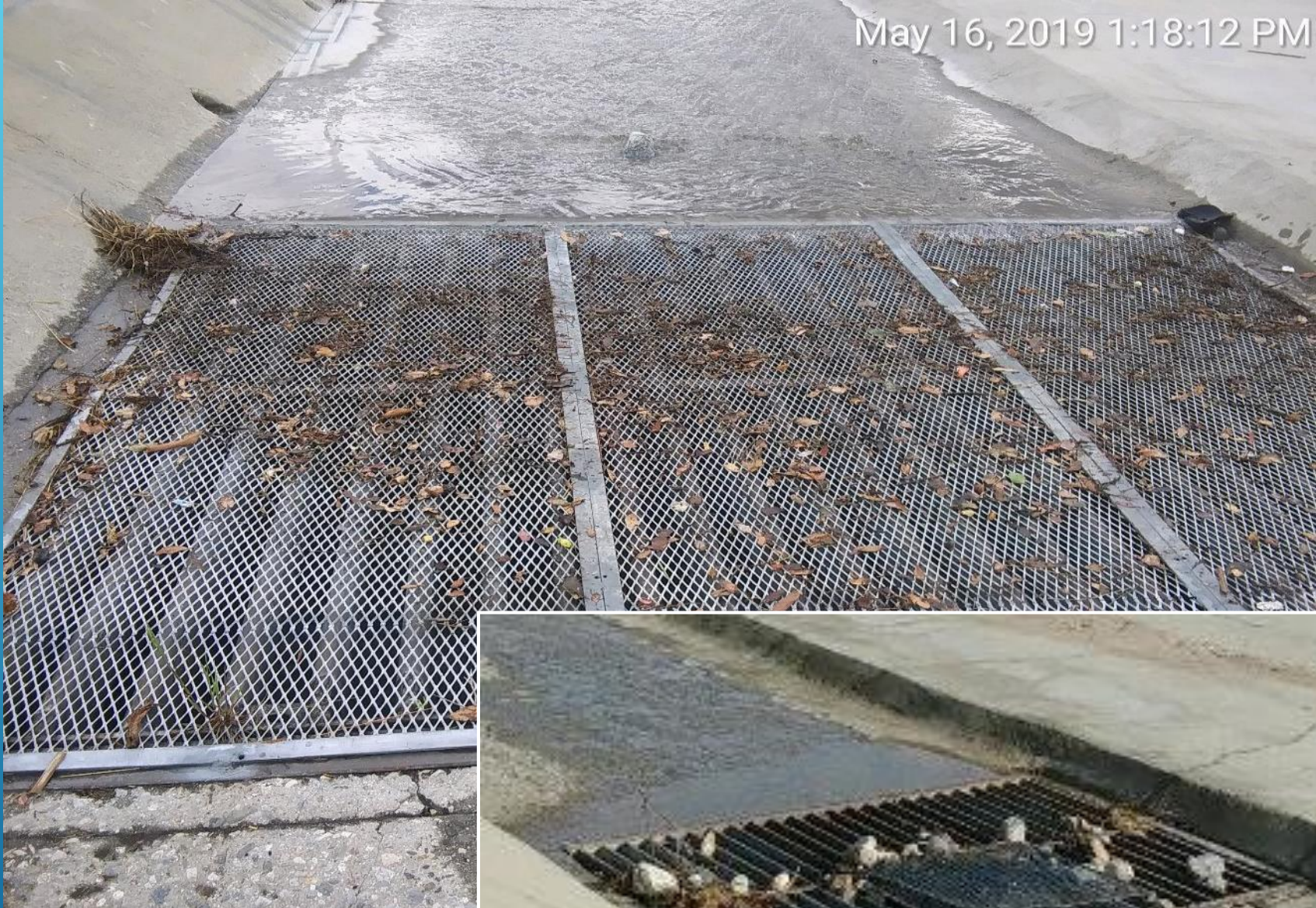
ETIWANDA INLET TO VICTORIA GRATE REPLACED (WELDED IN PLACE)
