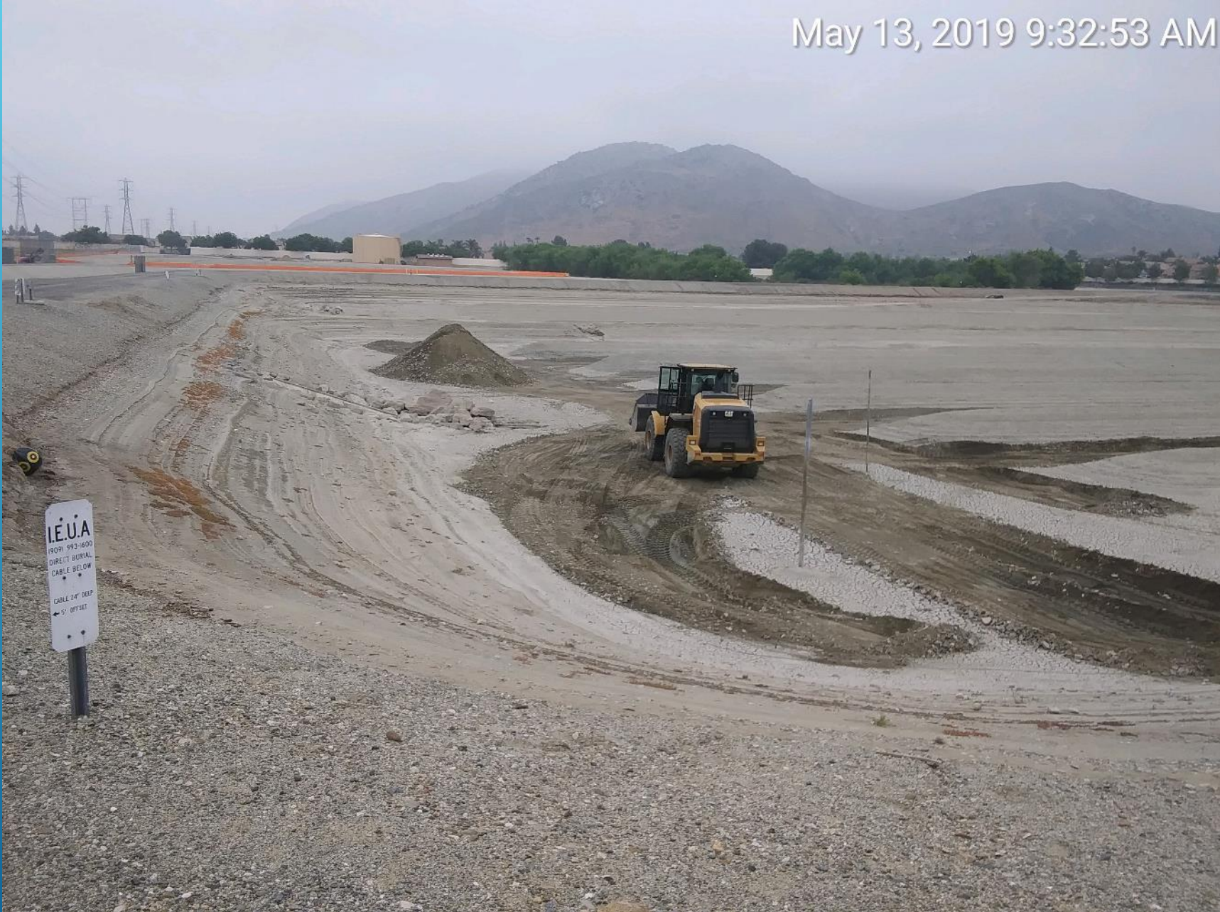
RP3 BASIN Scraping Cell 3
