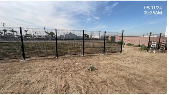
Welded Wire Mesh Steel Fencing
