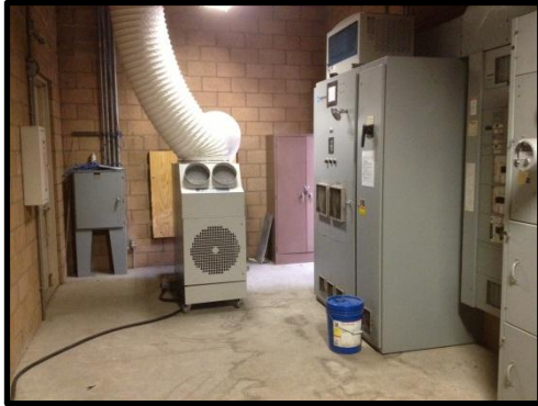
MCC Control Panel
