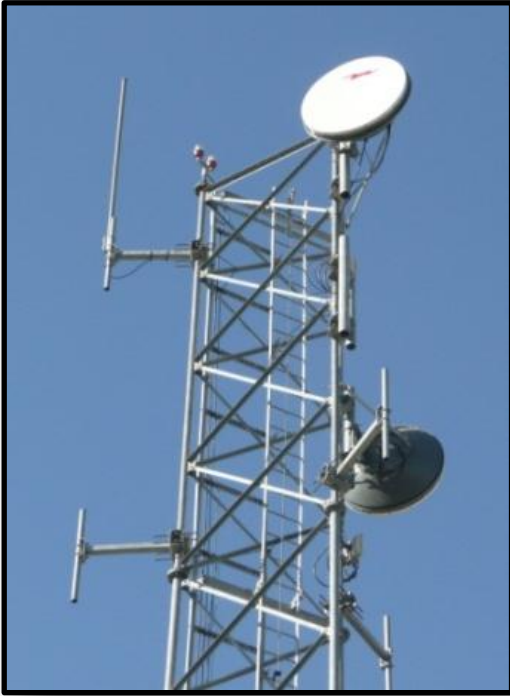
Basin Communication Tower
