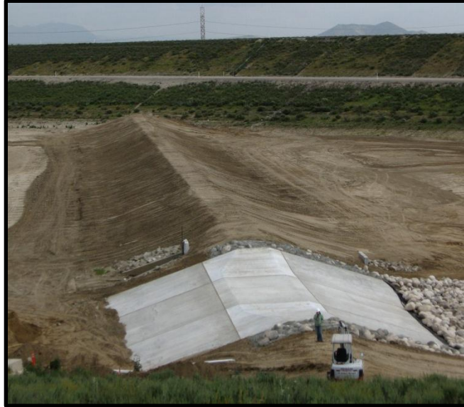
San Sevaine Basin 5 - Berm
