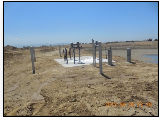
Completed Junction Structure with gates
