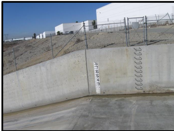
Berm removed and channel cleaned (12/03/13)
