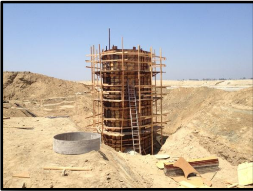
Construction of Junction Structure
