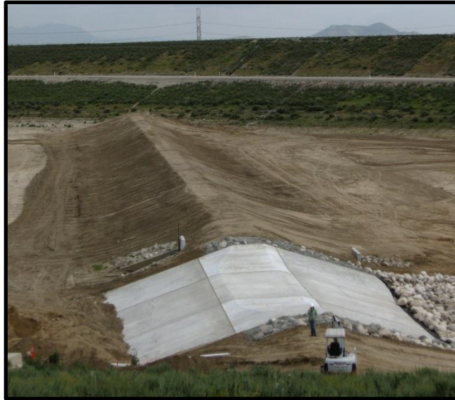
San Sevaine Basin 5 - Berm
