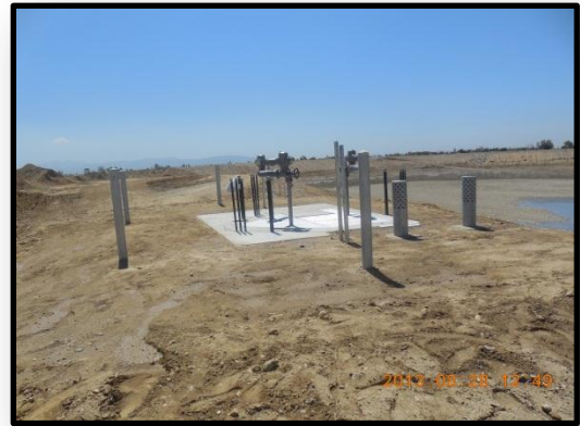
Completed Junction Structure with gates
