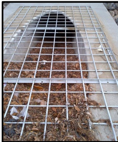
Installed 60-inch connection pipe into Basin 8 Junction Structure
