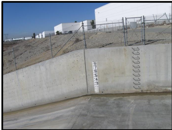
Berm removed and channel cleaned (12/03/13)
