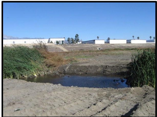
Access roads removed and basin restored to original (12/03/13)
