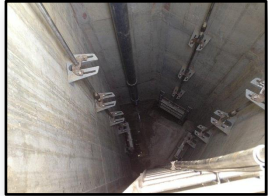
Inside the Completed Junction Structure
