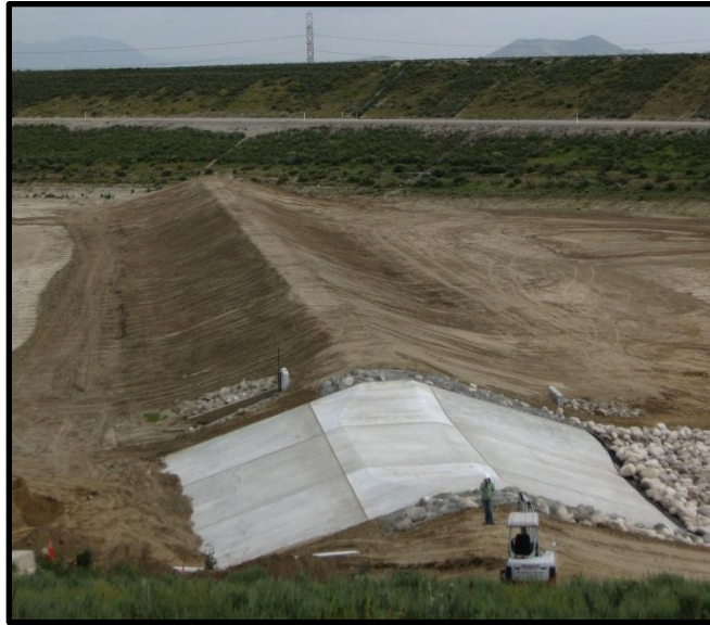
San Sevaine Basin 5 - Berm
