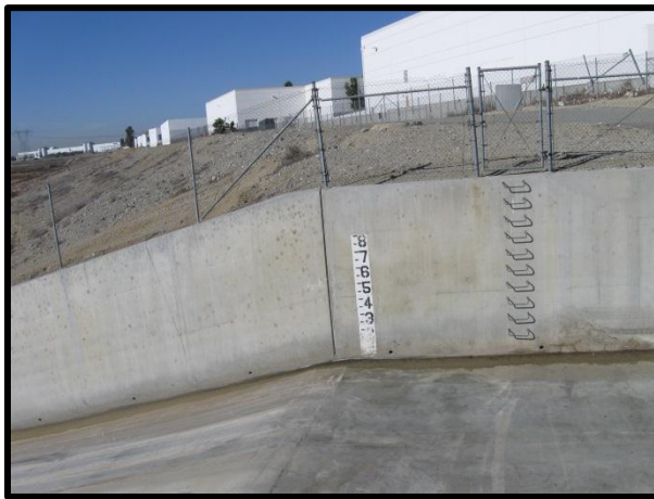
Berm removed and channel cleaned (12/03/13)
