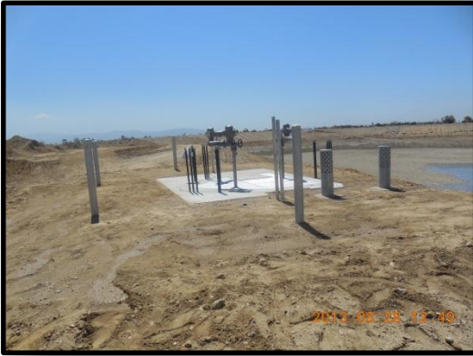
Construction of Junction Structure
