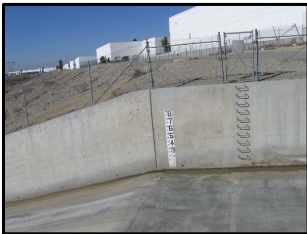
Berm removed and channel cleaned (12/03/13)
