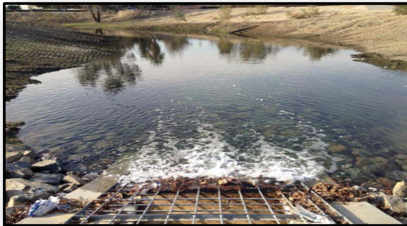
Installed 60-inch connection pipe into Basin 8 Junction Structure
