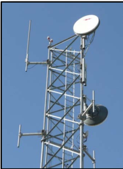
Basin Communication Tower
