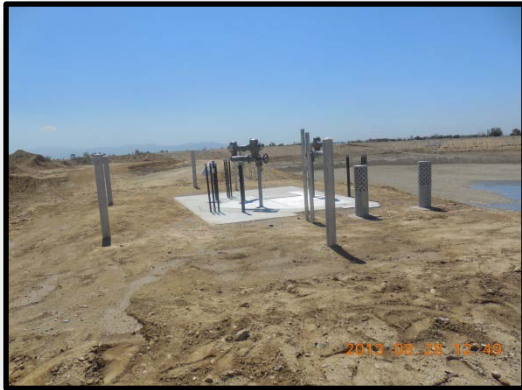
Construction of Junction Structure
