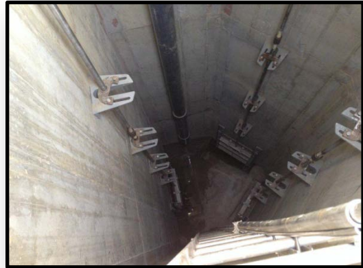
Inside the Completed Junction Structure
