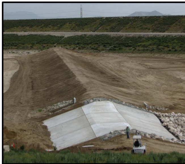
San Sevaine Basin 5 - Berm
