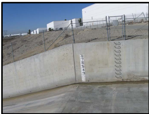
Berm removed and channel cleaned (12/03/13)
