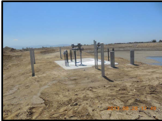
Construction of Junction Structure
