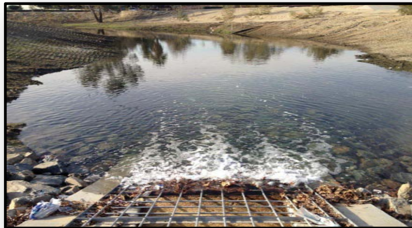
Installed 60-inch connection pipe into Basin No. 8 Junction Structure
