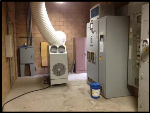
MCC Control Panel
