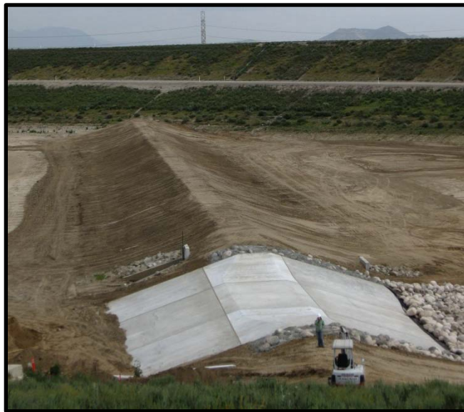
San Sevaine Basin 5 - Berm
