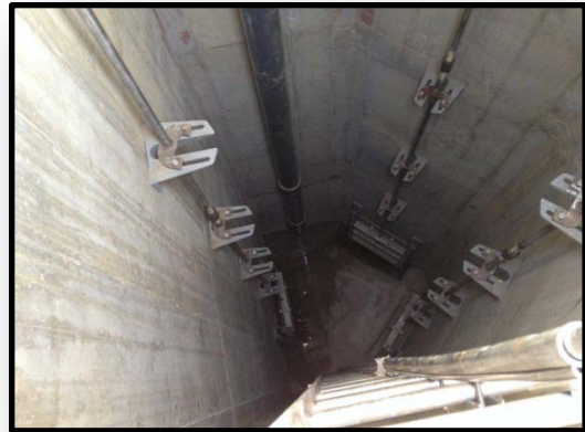
Inside the Completed Junction Structure
