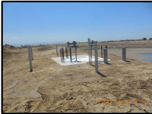
Construction of Junction Structure
