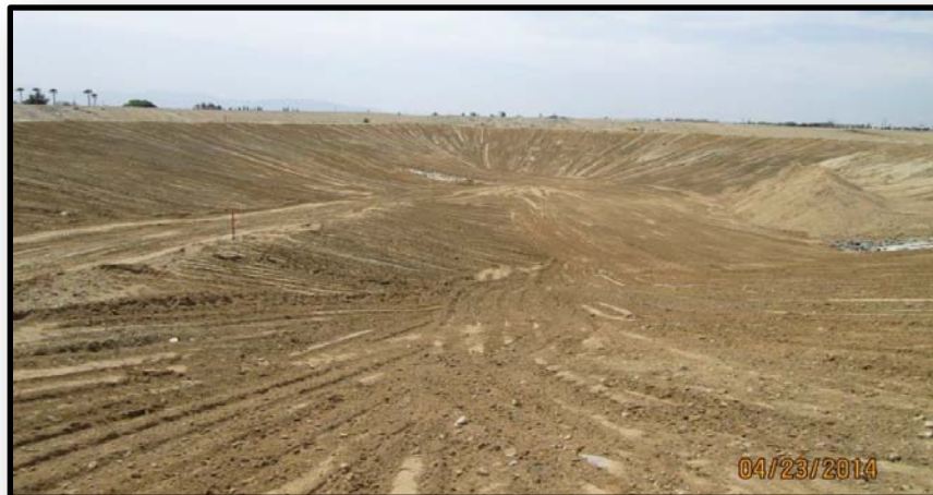
Completed new south basin
