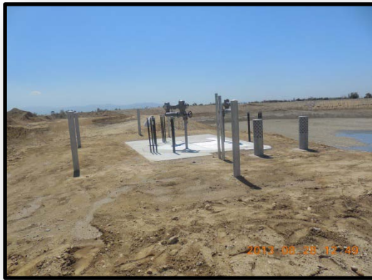
Completed Junction Structure
