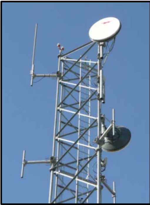
Basin Communication Tower
