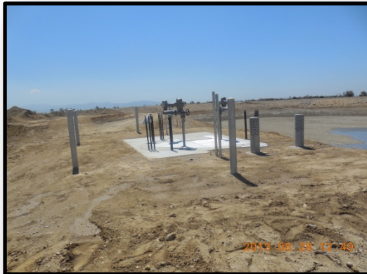
Completed Junction Structure
