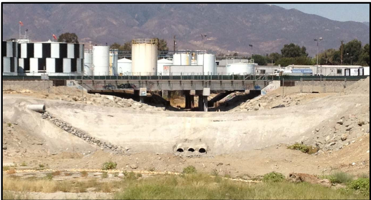
Completed Arizona Crossing which spans the inlet channel
