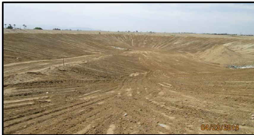
Completed new south basin
