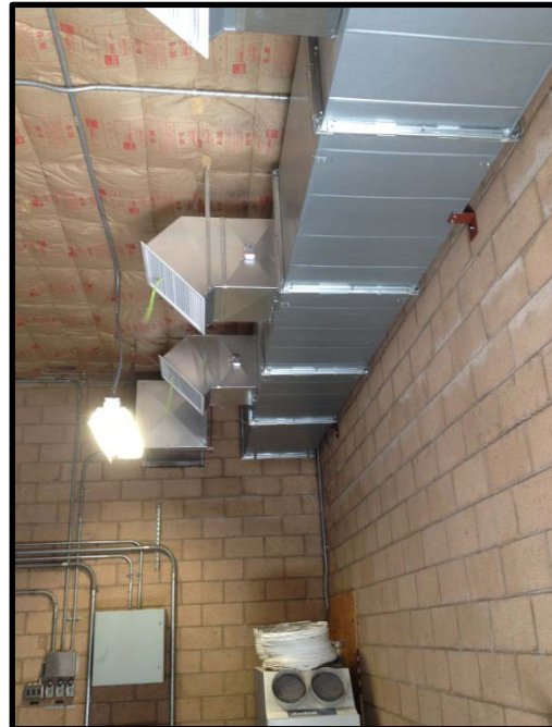
Installed ceiling Insulation and AC air ducting
