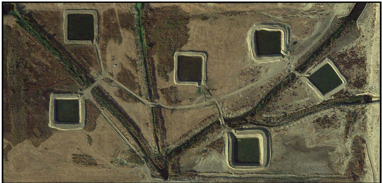
Figure 1- Temporary Infiltration Test Cells Constructed at Wineville
