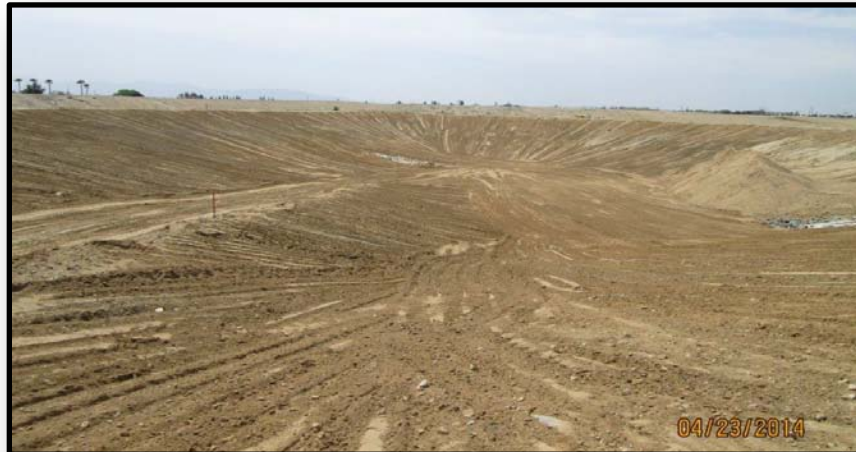
Completed new south basin
