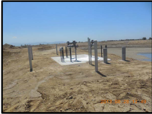
Completed junction structure
