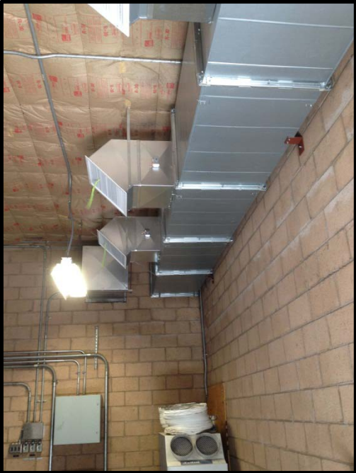
Installed ceiling insulation and AC air ducting
