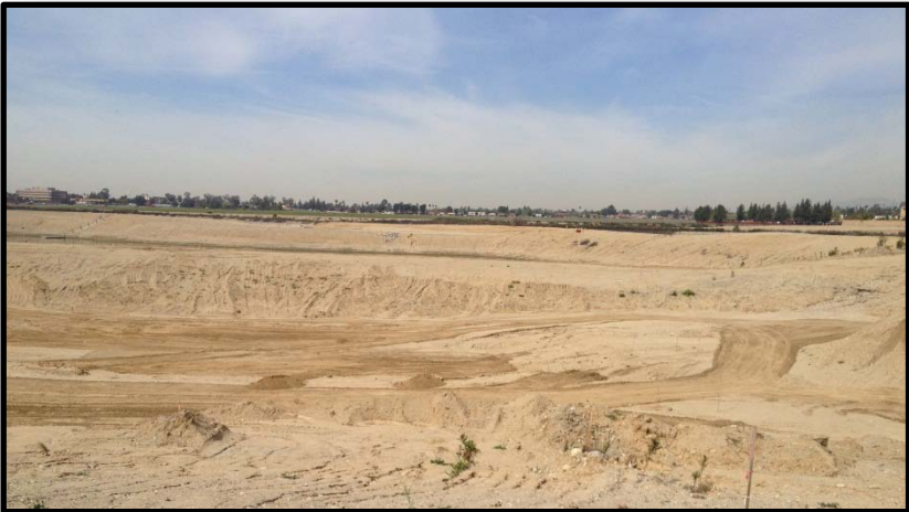
New north basin – grading/hauling in progress
