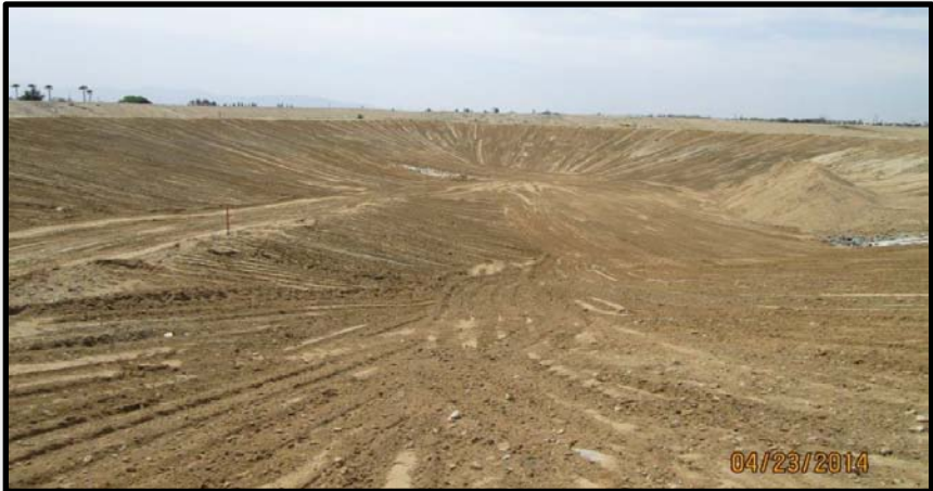
Completed new south basin
