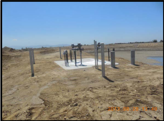
Completed junction structure
