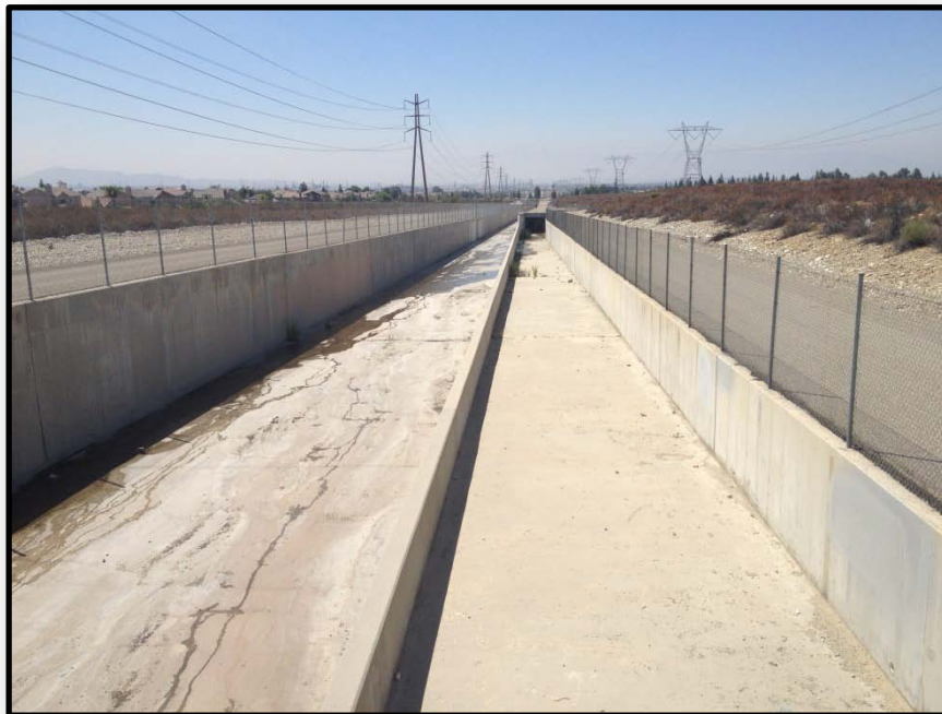
Field photo showing the location of the proposed improvement to the existing channel to increase storm water capture
