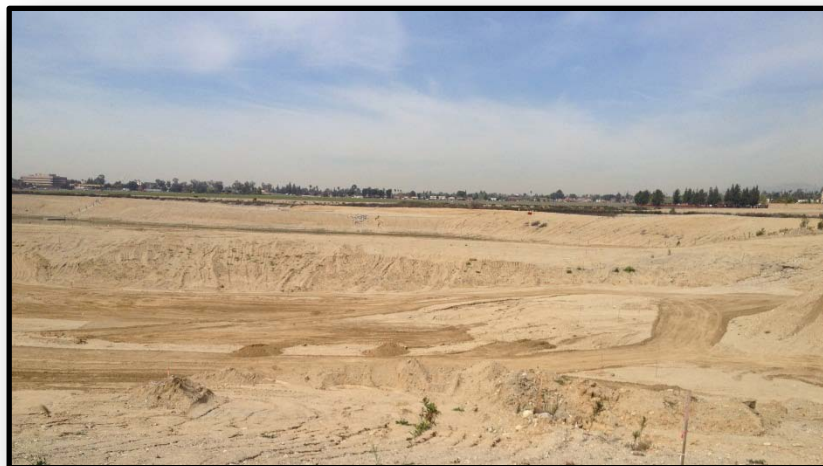
New north basin – grading/hauling in progress
