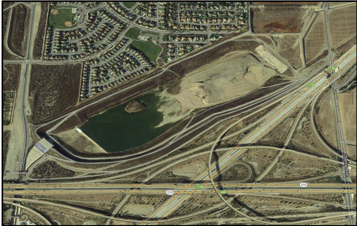
Aerial view of San Sevaine Basin No. 5
