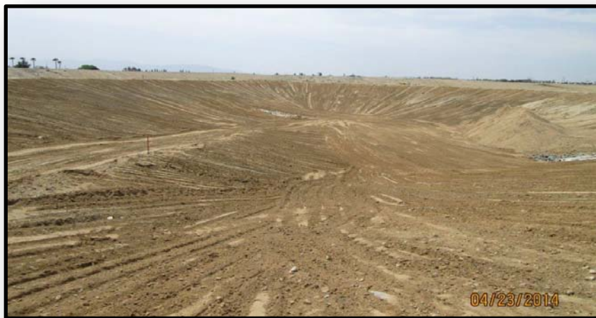
Completed new south basin
