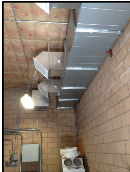
Installed ceiling insulation and AC air ducting
