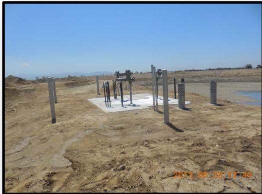
Completed junction structure
