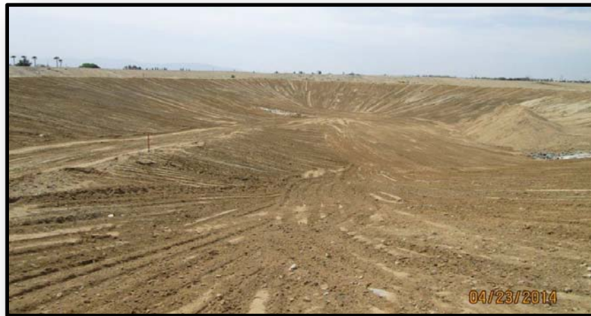
Completed new south basin
