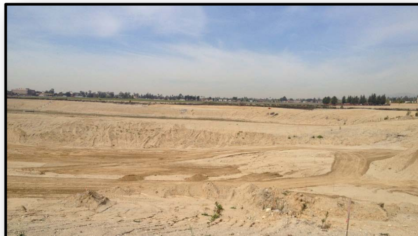
New north basin – grading/hauling in progress
