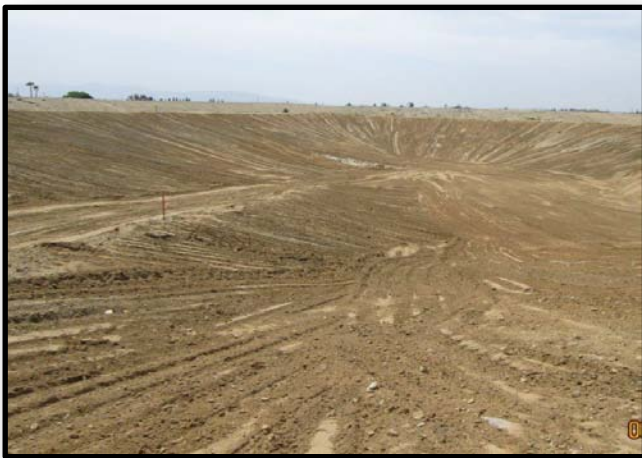
Completed new south basin (Turner 4c)
