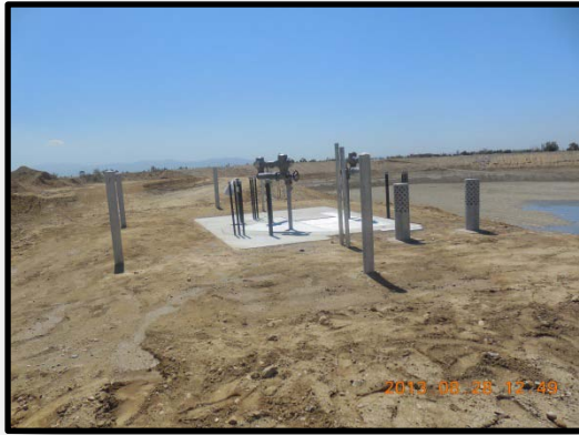
Completed junction structure
