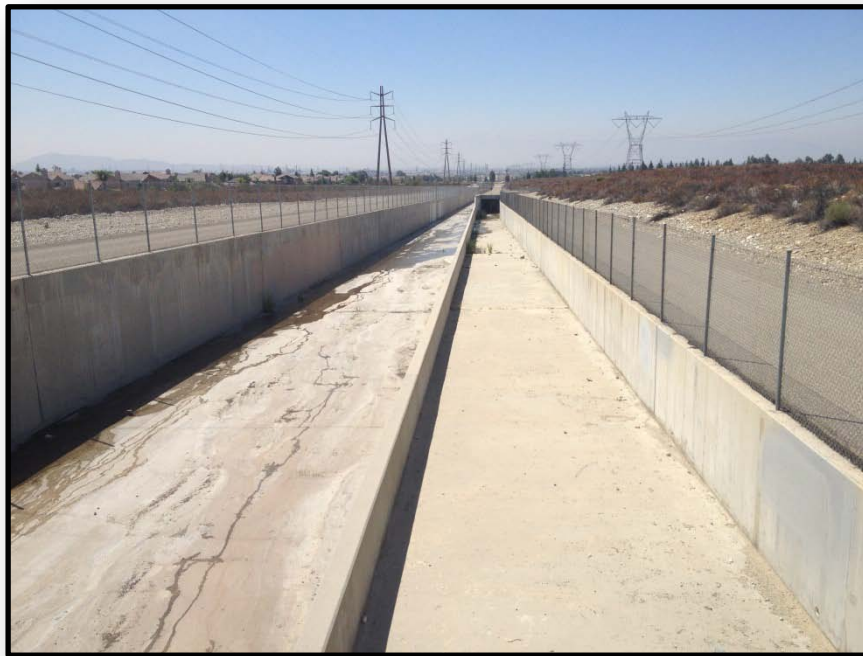
Field photo showing the location of the proposed improvement to the existing channel to increase storm water capture
