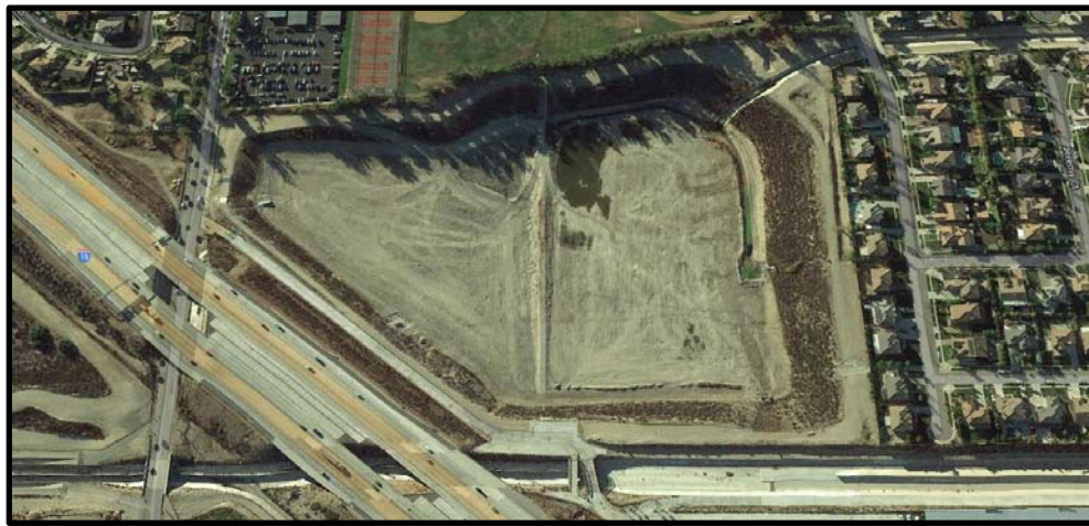
Aerial of Victoria Basin
