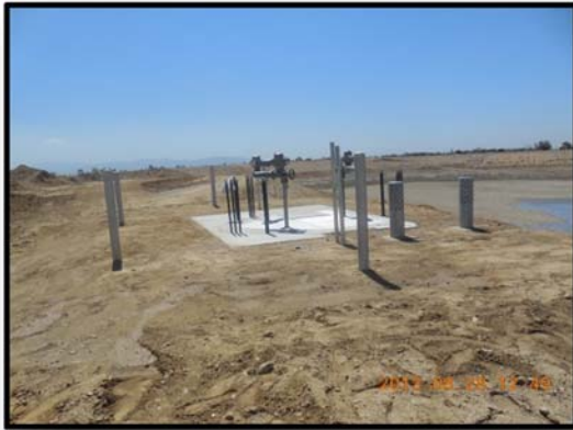
Completed junction structure
