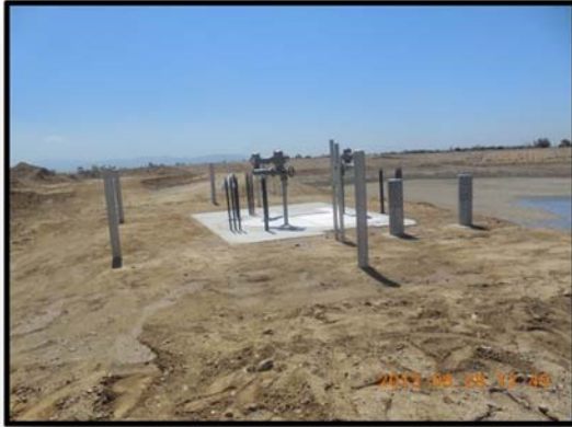
Completed junction structure
