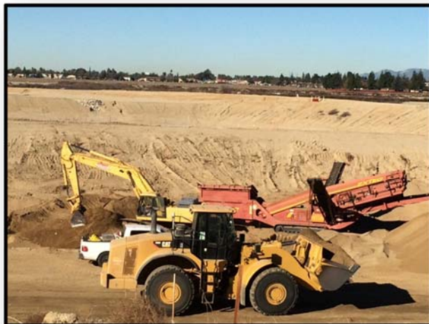
New north basin (Turner 4b) – grading/hauling in progress
