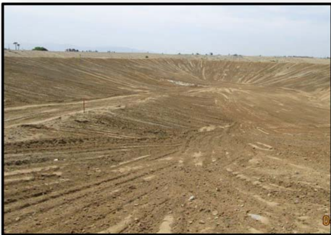
Completed new south basin (Turner 4c)
