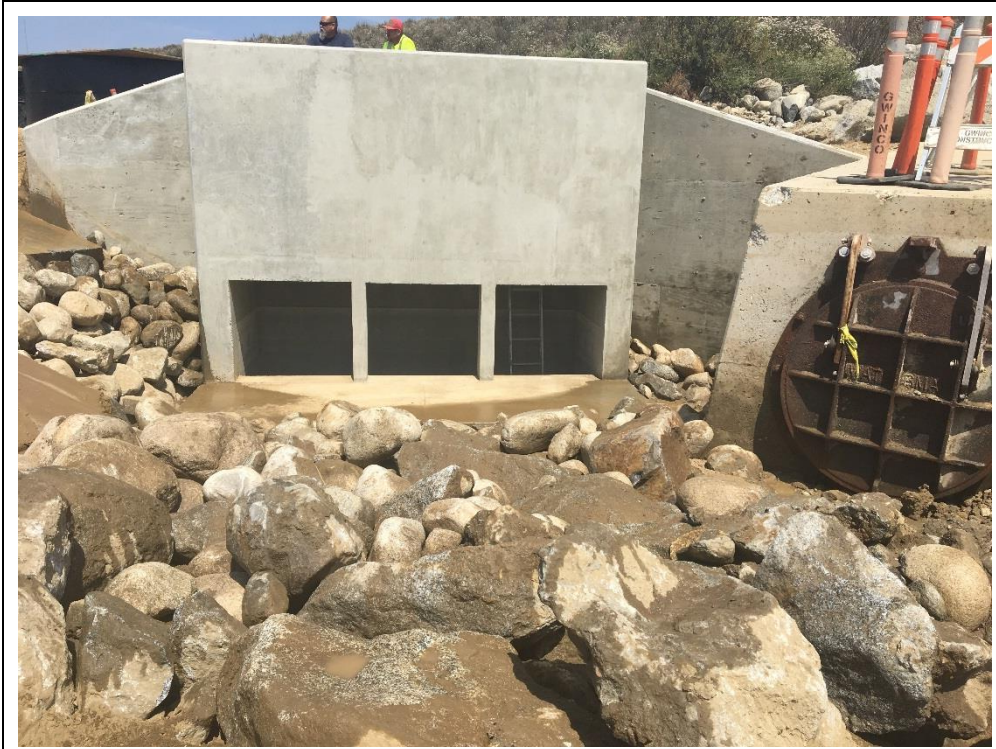
Storm water inlet structure
